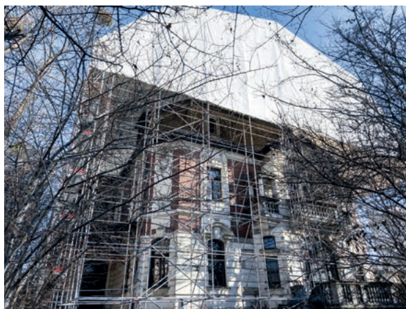
High wind exposure on the eaves side and highly structured architecture prompted the decision to use standard Allround scaffolding parts for simple and flexible adaptation to building geometry.
