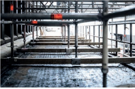
Due to its unclear structural properties, the hot alley was not allowed to be used to reduce the total weight on the scaffold.
