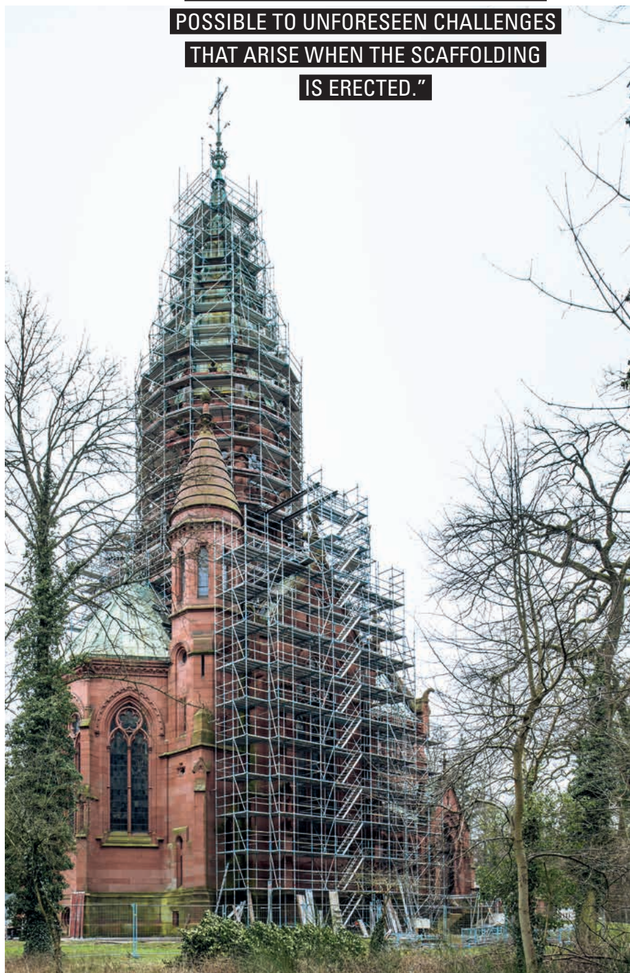
The tower needs to be refurbished first, before the typical sandstone facade of the church itself. Initially, therefore, the lower sections are only designed as shoring for the actual work scaffolding around the tower.
