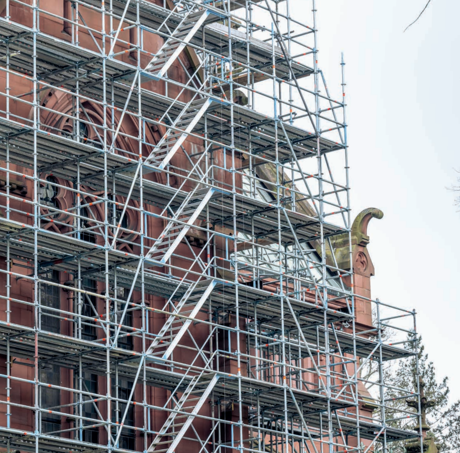
The facade scaffolding at the rear of the sepulchral chapel with stairway access
