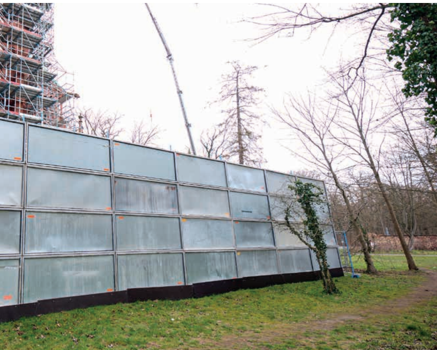
A Layher Protect System enclosure protects the construction site against unauthorised access.
