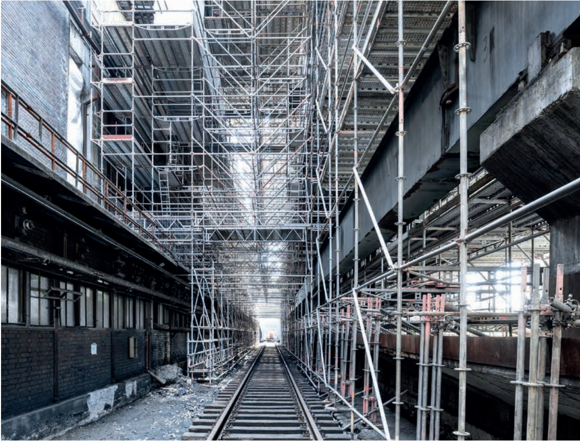
An 8,000 m 3 birdcage scaffolding element inside the hall provides the team of refurbishers with easy and safe access.
