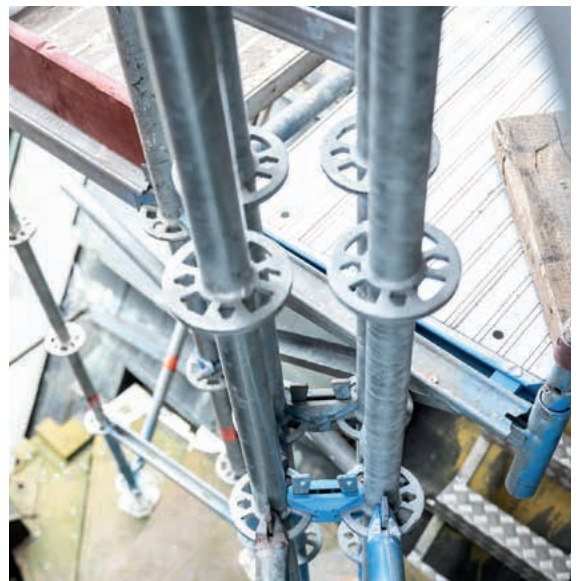
The steel beams for reducing the total weight on the work scaffolding are likewise supported on the load-bearing structures made from Allround Scaffolding.
