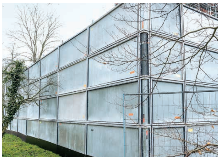
The Layher Protect cassettes can be quickly assembled on Allround Scaffolding.
