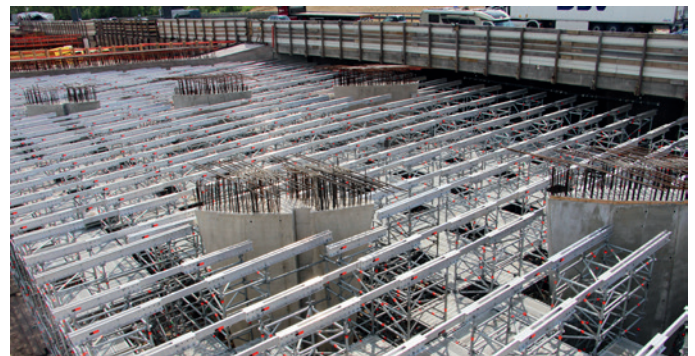
Fully assembled and calibrated shoring
